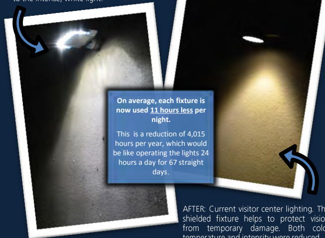
BEFORE: Previous visitor center lighting. Note both the glare emanating from the fixture and the amount of insects on the wall drawn to the intense, white light.
