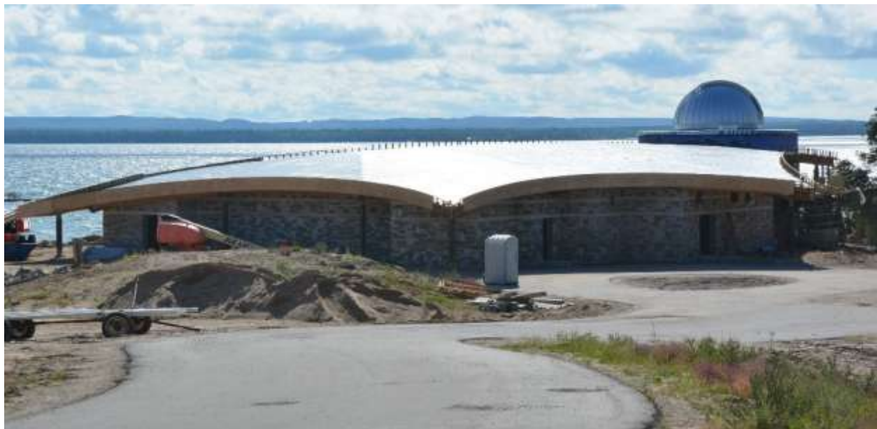
Clockwise from top left ~ construction site February 2016; drone's-eye view, September 2016; looking west toward Headlands Waterfront Event Center and Observatory where green roof is being prepped, September 2016
