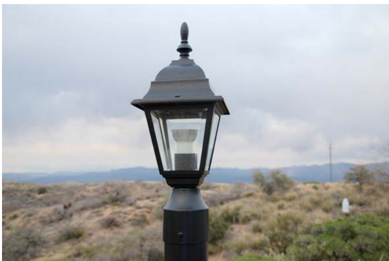
Figure 3.5 Amber LED style bulbs installed in March 2015
