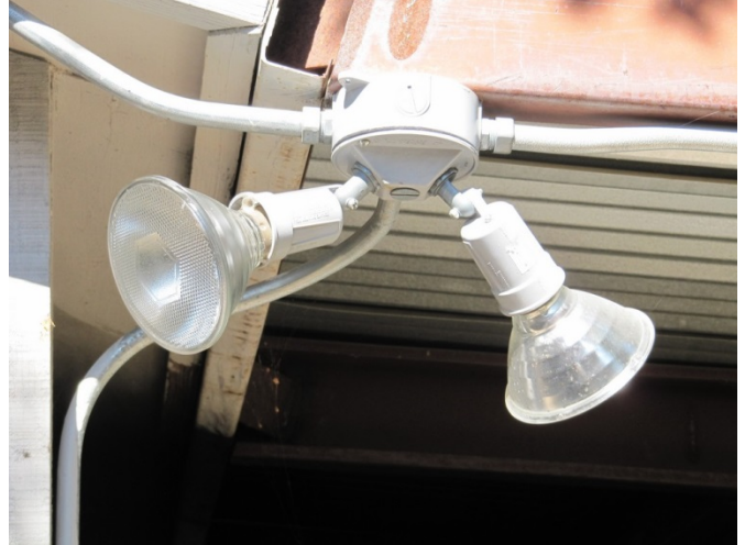
Cooler 1 Photograph Reference: CS-4
