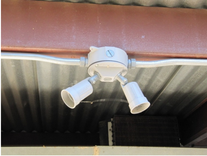
Cooler 2 Photograph Reference: CS-5
