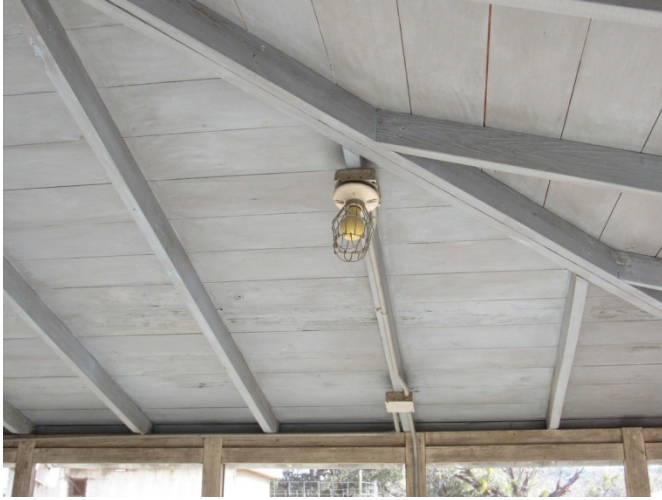
Screened in porch Photograph Reference: HQ-1
