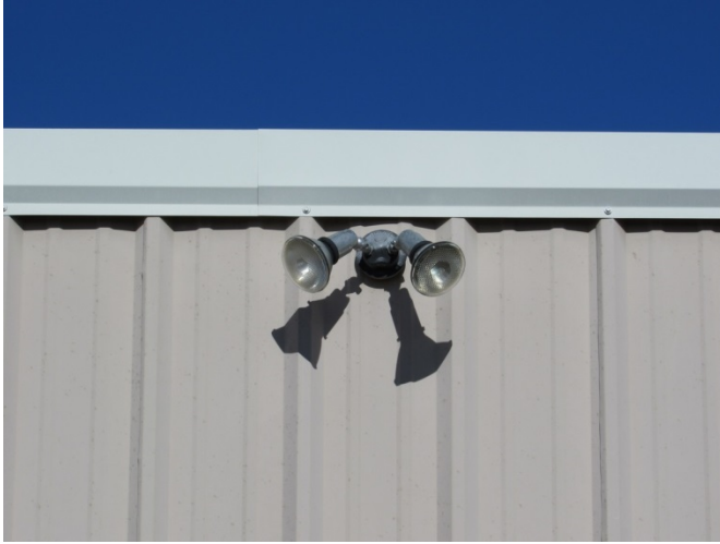
Garage South Photograph Reference: CS-9
