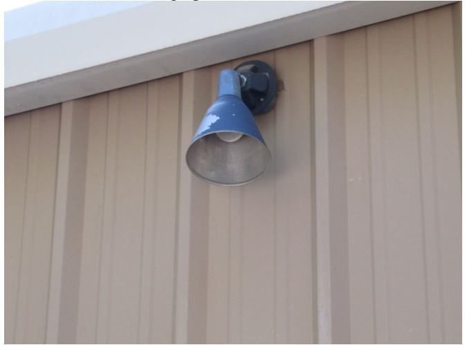
Garage North 2 Photograph Reference: CS-8
