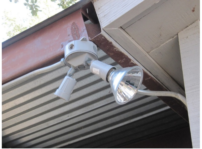
Cooler 3 Photograph Reference: CS-6
