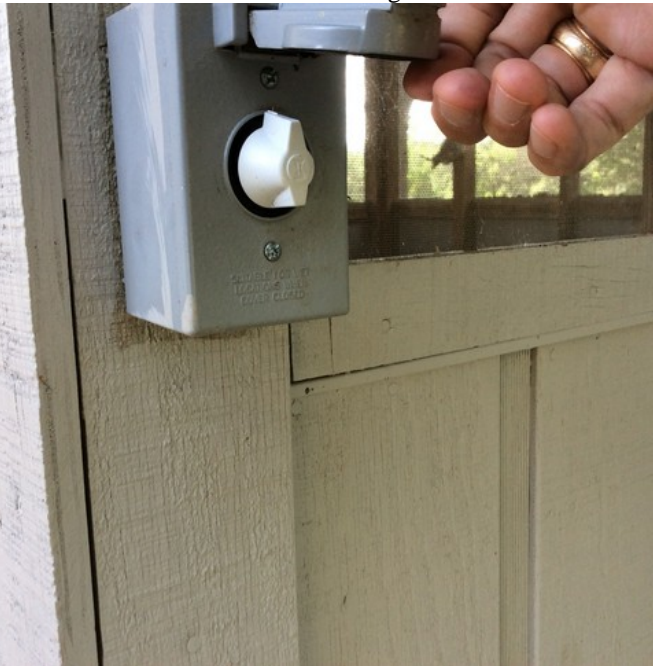
Timer Switches Outdoor floodlights
