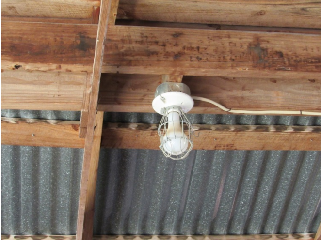
Inside Barn Ceiling Lighting Photograph Reference: HQ-5
