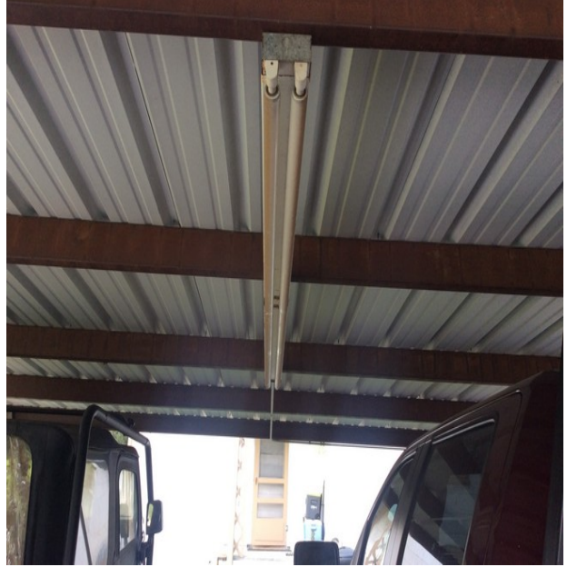
Carport Photograph Reference: AM-2
