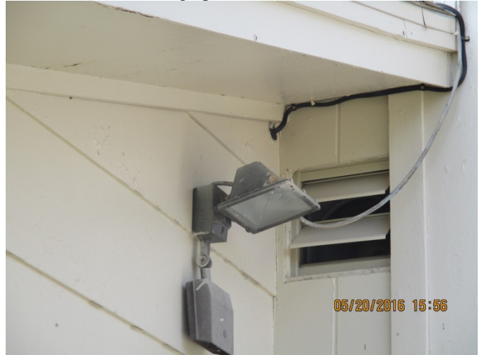
Outside Light East Photograph Reference SH-2
