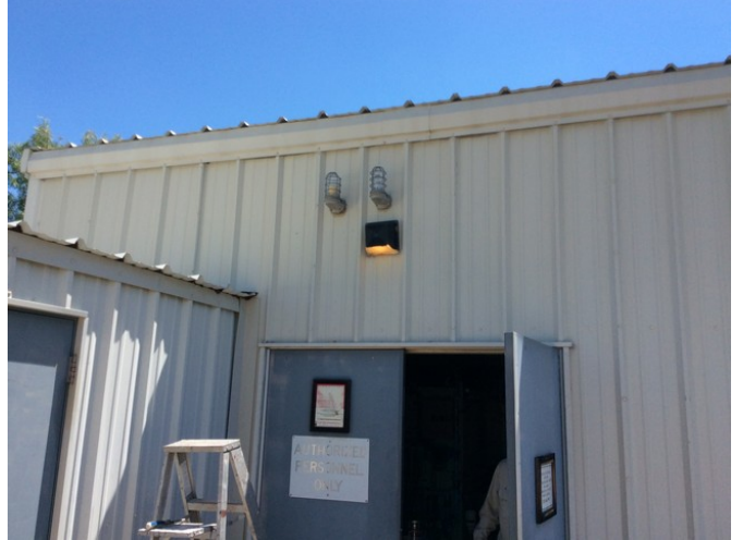
Water Treatment Plant Entrance Emergency Lights (After) Photograph Reference: M-4
