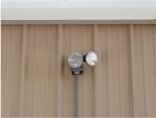
Garage North 1 Photograph Reference: CS-7
