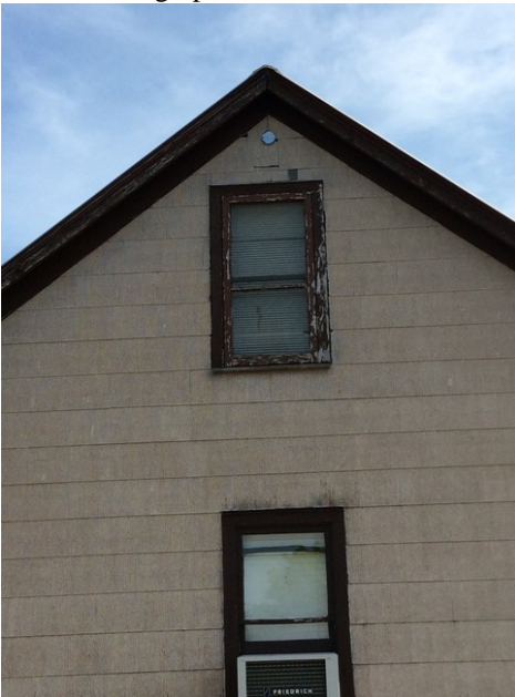
Cabin North (After Removal) Photograph Reference: HC-2
