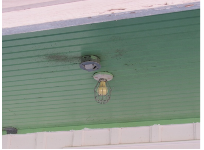
Front Porch Photograph Reference: HQ-6
