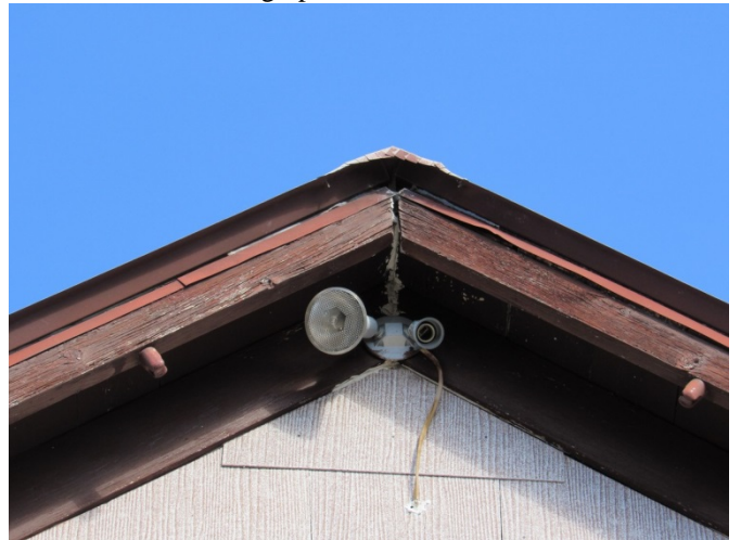
Cabin South (Before) Photograph Reference: HC-3
