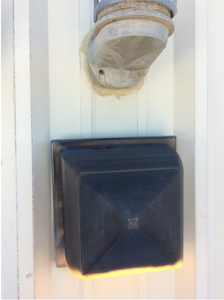
Water Treatment Plant Entrance Emergency Lights (After) Photograph Reference: M-4
