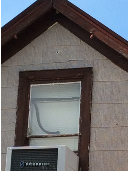
Cabin South (After Removal) Photograph Reference: HC-3
