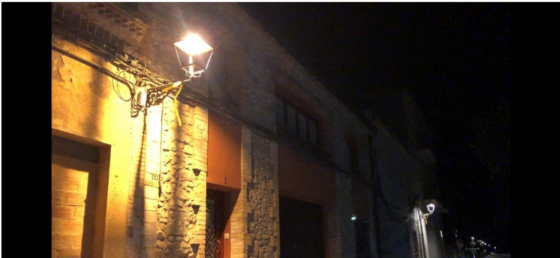
Pilot testing of 2700K LED lighting.
