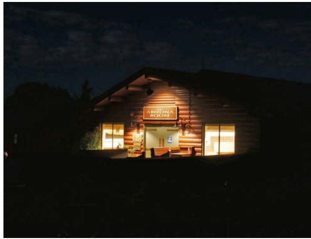
Arizona Room after retrofit
