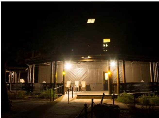
El Tovar North Porch before retrofit
