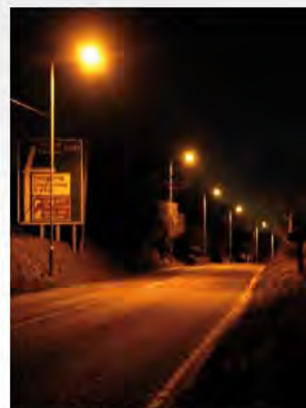
Lighting on A487 extending into the open countryside
