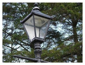
**Figure 2.13: Good example of Heritage Luminaire** with rear light limiter, lamp recessed in canopy hood and light distribution using pot-optic.
