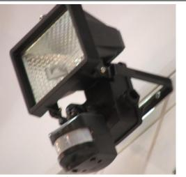
**Poor** – Lamp reflector and PIR detector point in same elevation and rotational direction. 300 / 500 watts Tungsten Halogen lamps provide too much light for use in rural settings.
