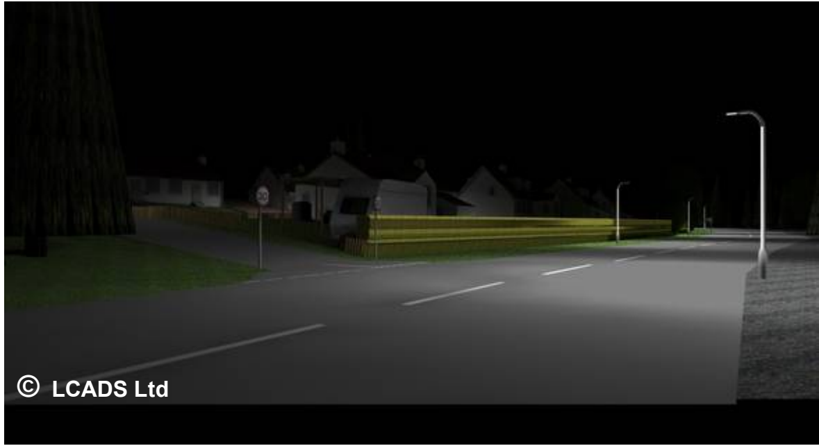
Figure 1.7 Luminaires with Fully Shielded distribution showing distinct lack of upward spill light detail and distinct reduction in distant visual glare from the luminaires.
