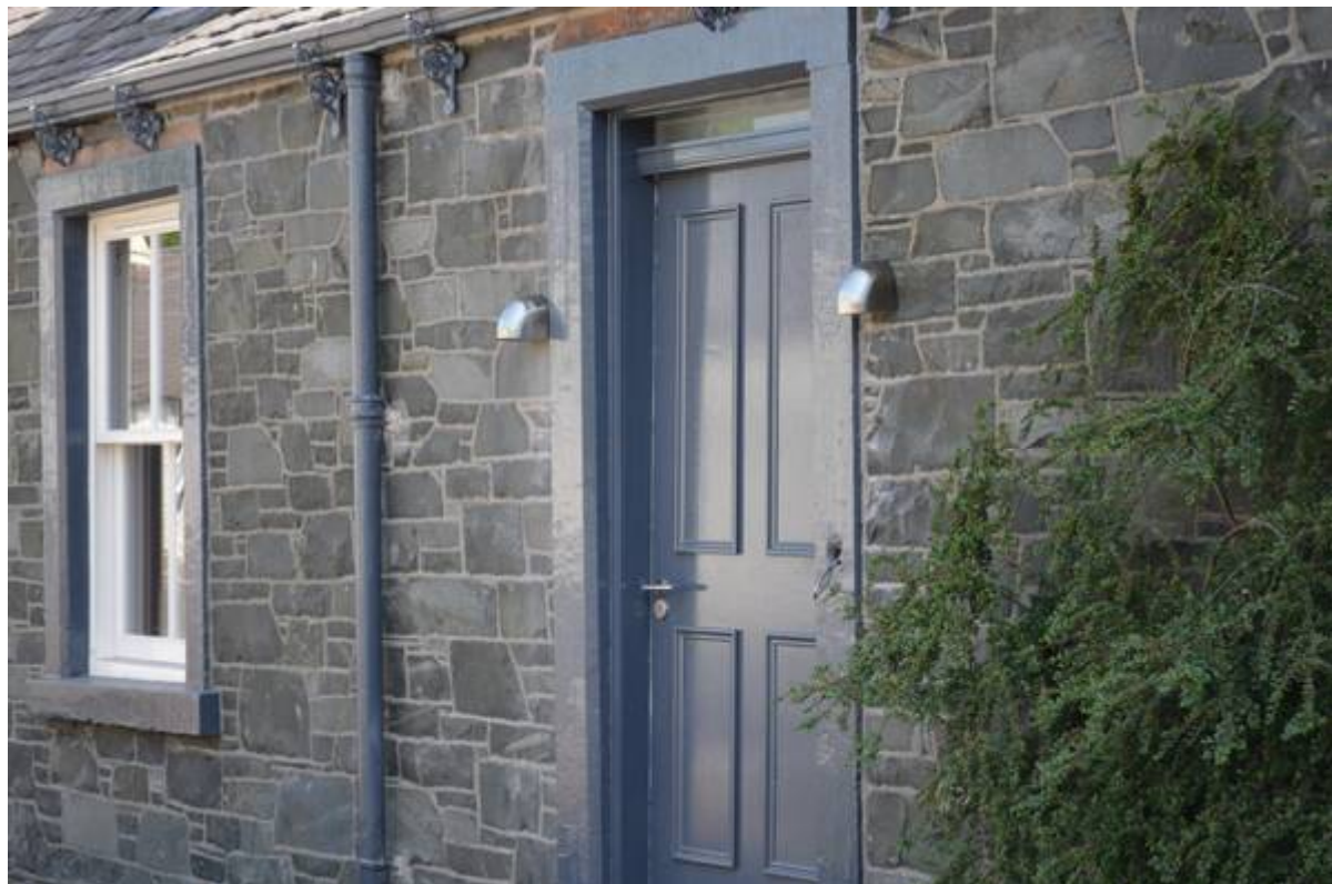
Figure 5.8 Example of new door lights installed during house renovation in Holm Street
