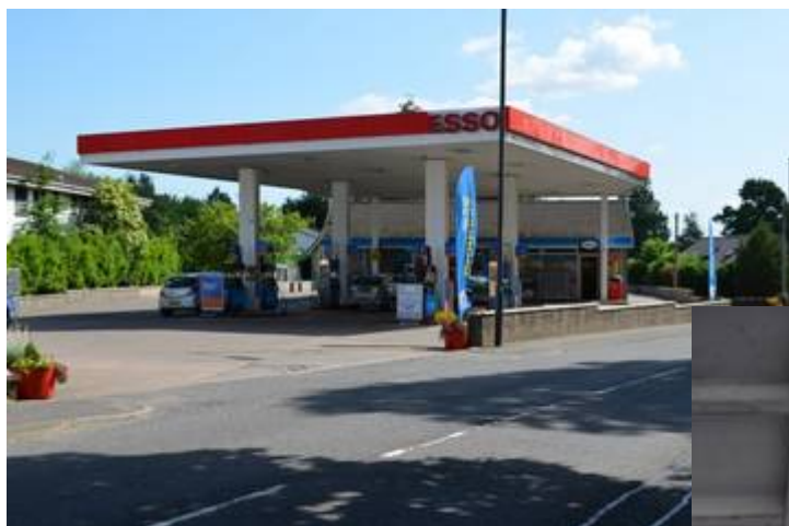
Figure 5.7.1 Petrol Filling Station
