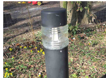
Figure F.1: NonFCO, clear glass, UH: 41% UL: 9% ULR: 50%.
