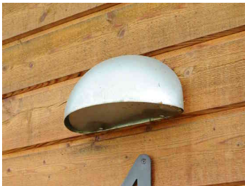
Figure E.7: FCO, frosted glass. UH: 0%, UL: 0%. This type fixture is populaer among the companies with the local Dark Sky Certification.
