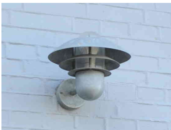
Figure E.9: NonFCO, clear glass, UH: 15 - 35% de- pending on the installed light source. UL: <5% ULR: 15 - 40%
