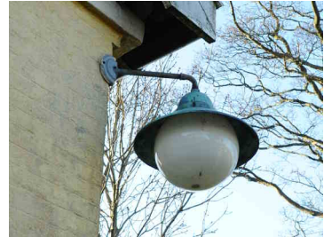
Figure E.35: Rar historic fixture, nonFCO, frosted glass, UH: 5% UL: 9%, ULR: 14%
