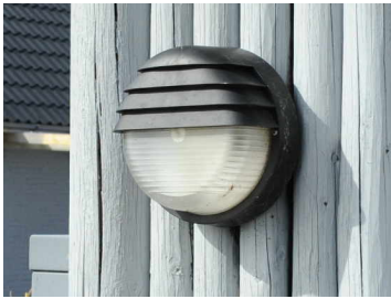
Figure E.4: NonFCO, textured plastic, UH: 10-15%, UL:5-10%, ULR: 15-20%
