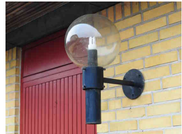
Figure E.23: This is a really complicated fixture just to show of a bare light bulb, but unfortunately these types of fixtures do exist! Absolute nonFCO. UH: 41%, UL: 9%, ULR: 50%.
