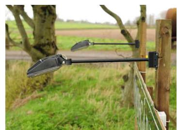
Figure E.27: Downlights for sign. Installed correct, as here, these fixtures are FCO. UH: 0%, UL: 0%, ULR: 0%
