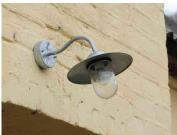
Figure E.18: NonFCO, clear glass. This fixture comes in two version. The version in the figure is angled approximately 25° upward, UH: 30 - 35% UL: 8 - 10%, ULR: 38 - 45%. The other version is angled down, UH: 20 - 25% UL: 8 - 10%, ULR: 28 - 35%
