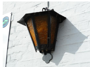
Figure E.2: NonFCO, yellow and textured glass. Fixture is not FCO and there is at possibility of glare, due to the yellow glass the CCT is very low, therefore it is accepted.
