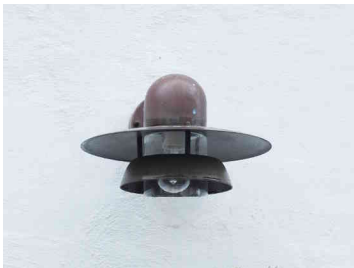
Figure E.19: With correct light source, as installed here, this is a FCO fixture. If wrong light bulb is used: UH: 0%, UL: <5%, ULR:<5%.
