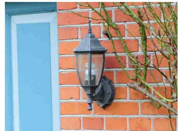
Figure E.37: NonFCO, frosted glass, UH: <10% UL: 9%, ULR: 15-19%
