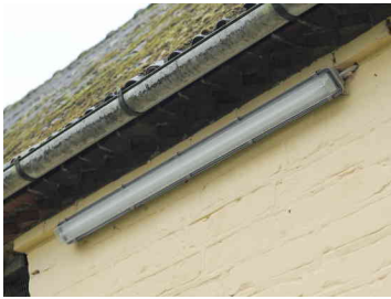
Figure E.16: In the figure the fixture is angled approximately 45° from horizontal. It is possible to find this kind of fixture installed in any angle from horizontal (0°) to 90°. Due to the different angles of installation the fixtures ULR varies considerably. UH: <10 - 41%, UL: 5 - 9%, ULR: <15 - 50%.
