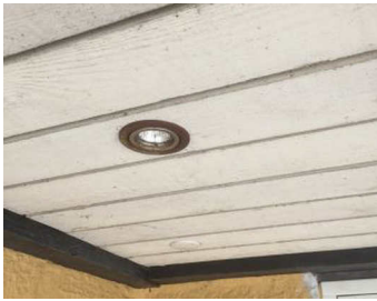
Figure E.40: FCO, mounted in ceiling, UH: 0% UL: 0%, ULR: 0%
