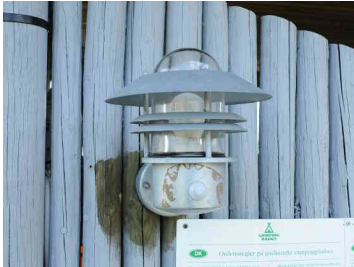
Figure E.5: NonFCO, clear glass, UH: 15 - 35% de- pending on the installed light source. UL: 5 - 10% ULR: 20 - 45%
