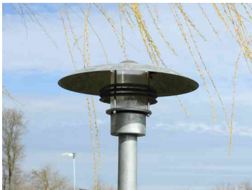
Figure E.6: NonFCO, clear glass, UH: 15 - 35% de- pending on the installed light source. UL: 5 - 10% ULR: 20 - 45%
