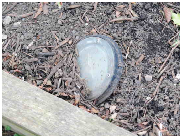
Figure E.30: Spotlight as uplight below a tree, non-FCO. UH: 100%, ULR: 100%.
