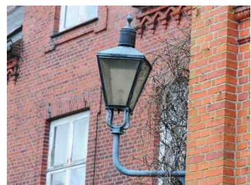
Figure E.39: NonFCO, frosted glass, UH: <10% UL: 9%, ULR: 15-19%
