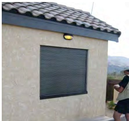
Partially shielded window illumination at west entrance
