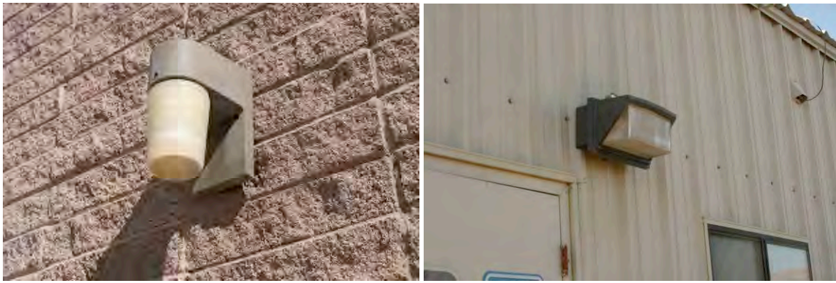
Figure 1a-b. Unshielded fixtures resulting in glare and light trespass.
