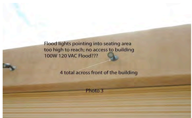
Indian Cove Stage lighting, should be pointed down
