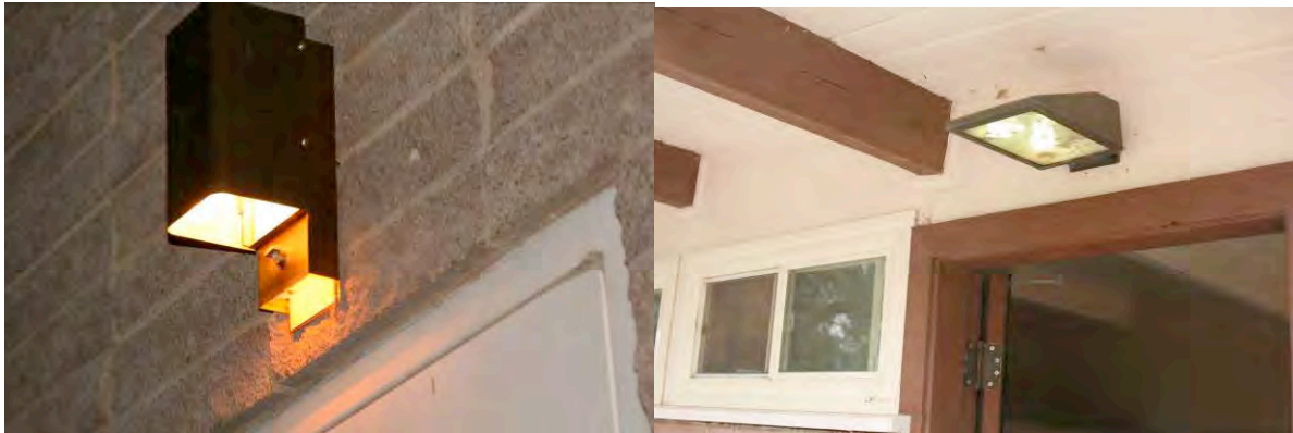
Figure 1a-b. Unshielded fixtures resulting in glare and light trespass.
