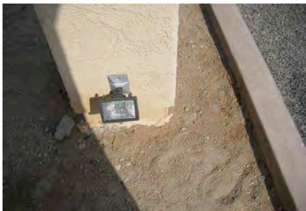
Upward pointing halogen flood at west entrance
