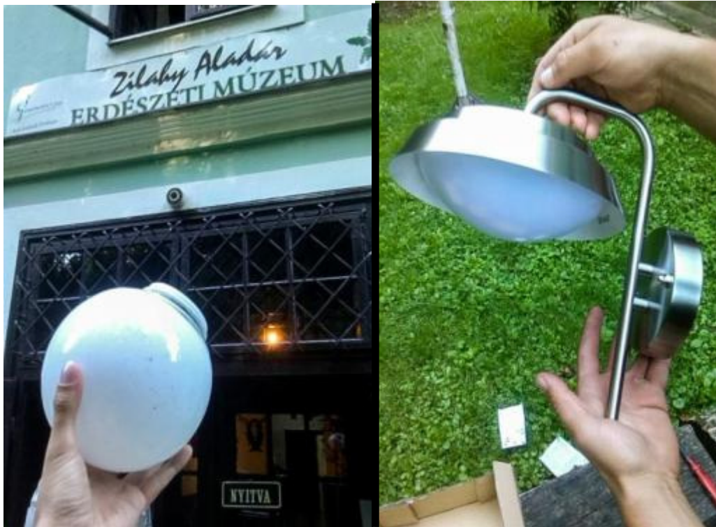
Replaced lighting fixtures in the Szalajka-valley
