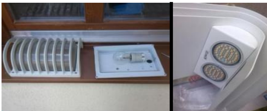
Old and new illuminators of the forest school walls made also for educational purposes (Field education center – Felsőtárkány)
