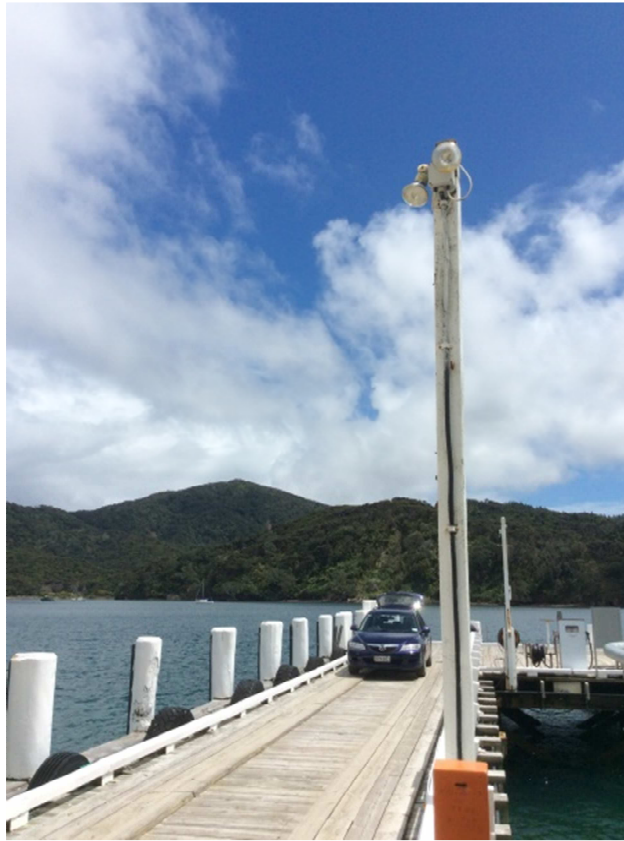
Above: Lighting at Whangaparapara Wharf, powered by generator and only used in emergencies
