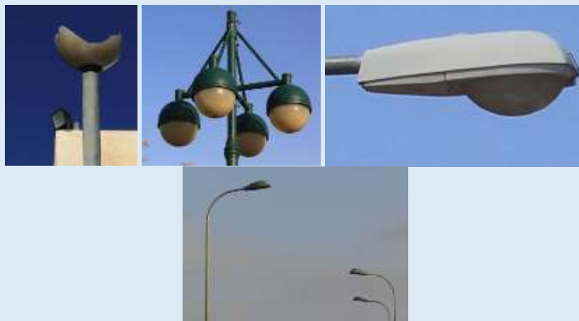
Fig 14: Bad and good (only the right!) oriented luminaires in Mitzpe Ramon
