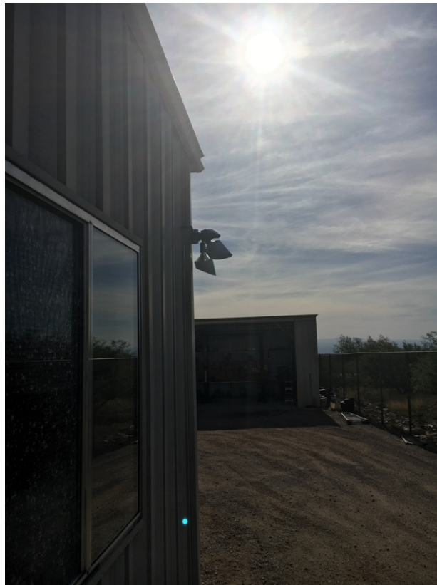
Figure 6.2 Light fixtures brought up to code
