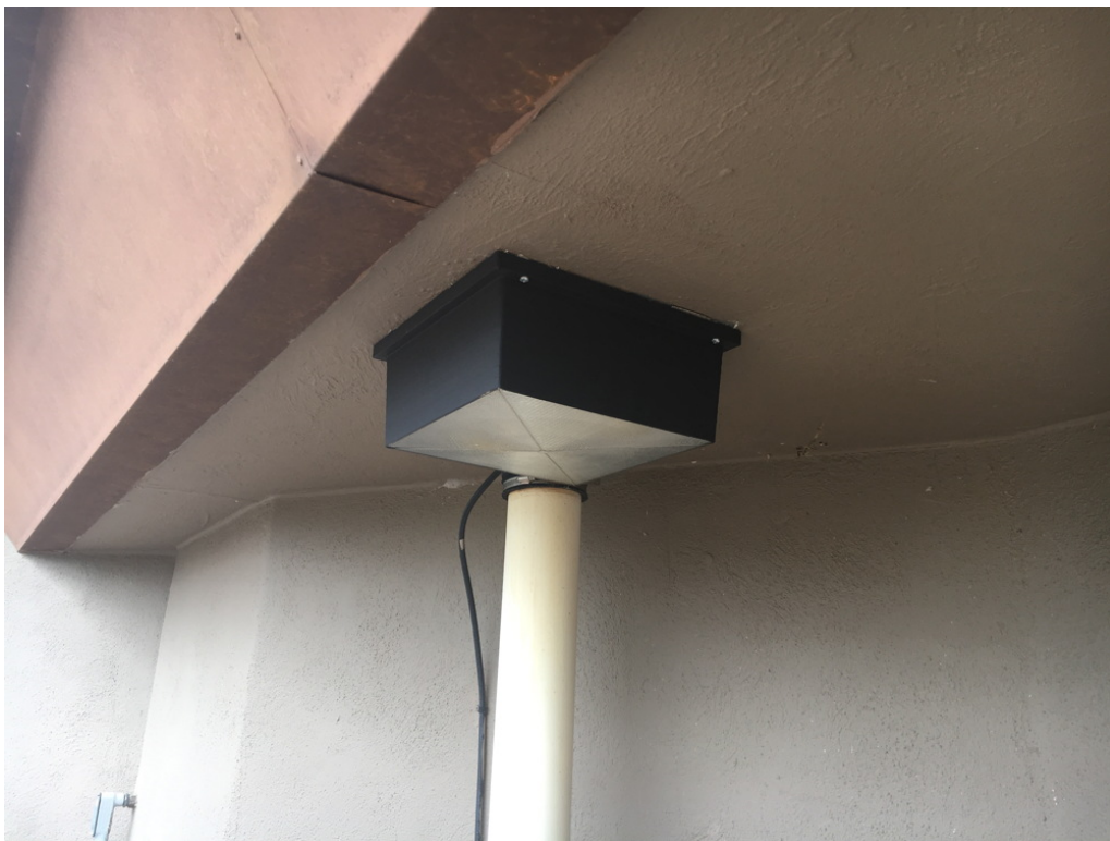
Figure 6.2 (continued) Light fixtures brought up to code
