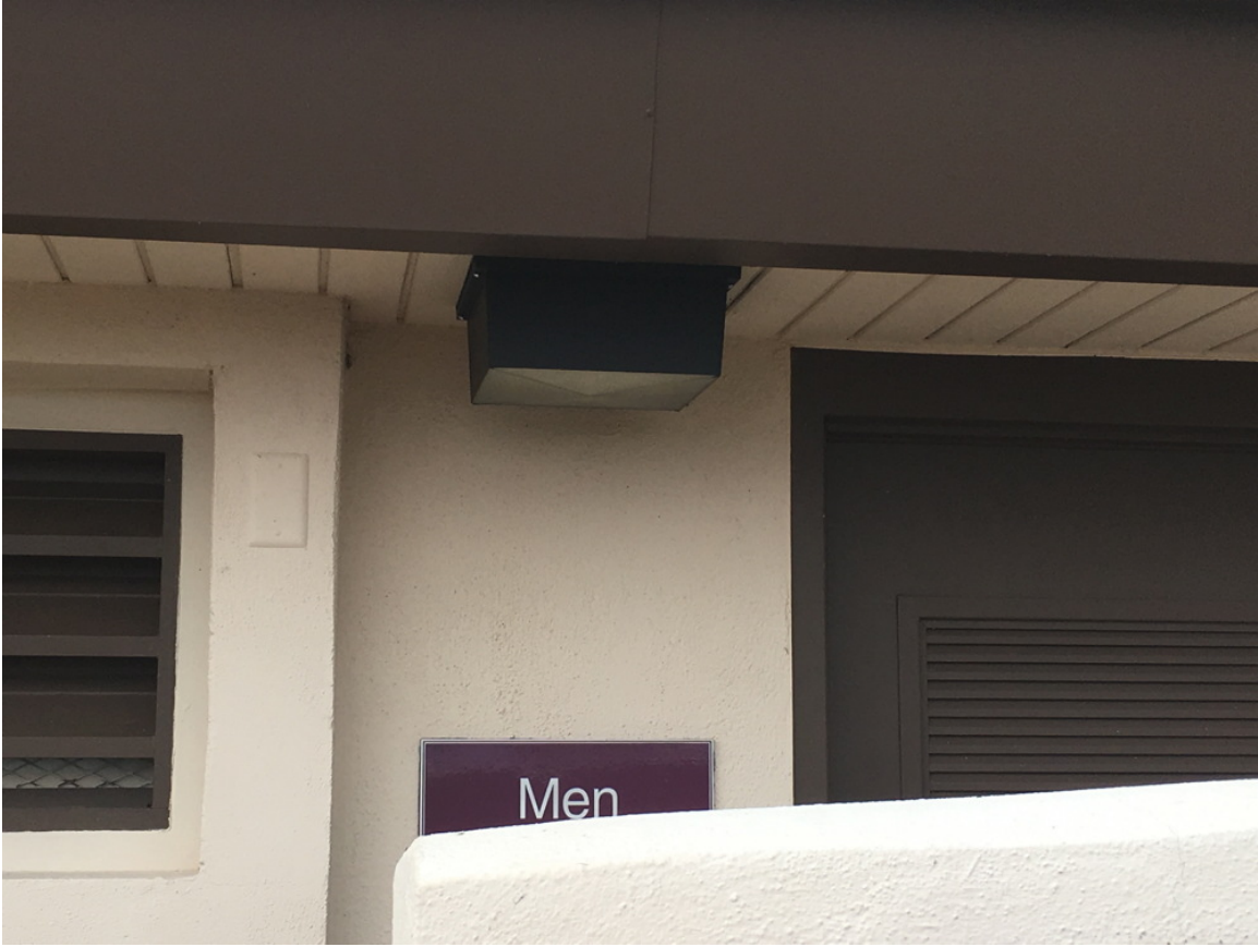
Figure 6.2 (continued) Light fixtures brought up to code
