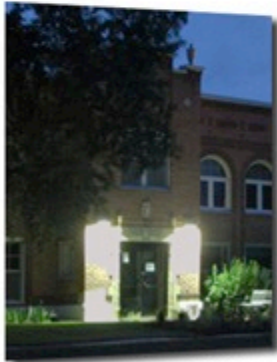
County Courthouse after— with shielded wall packs that direct lighting to the ground to provide safer entry
