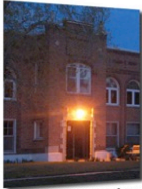
County Courthouse before— with glaring wall packs that blinded passing motorists
