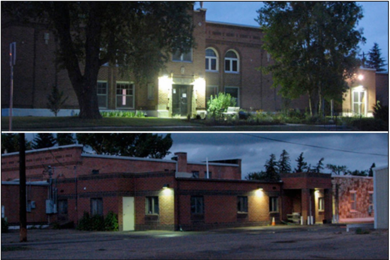
The top image is of the front of the Custer County Courthouse from Sixth Street/Highway 69 where the glaring wall packs used to blind passing drivers. The bottom image is the back of the courthouse where glaring wall packs were replaced (the shielded street lights in the parking lot are not shown).
