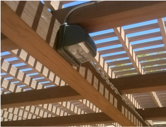
Figure 3-3. Before: High pressure sodium light at Pipe Spring National Monument Visitor Center
