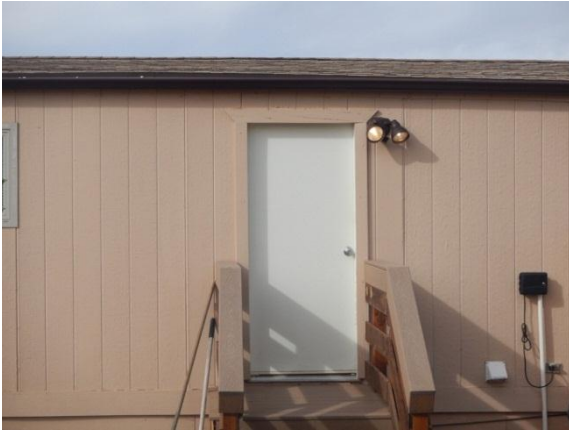
Figure 3-7. After: Motion triggered flood lighting retrofit at Pipe Spring National Monument Housing
