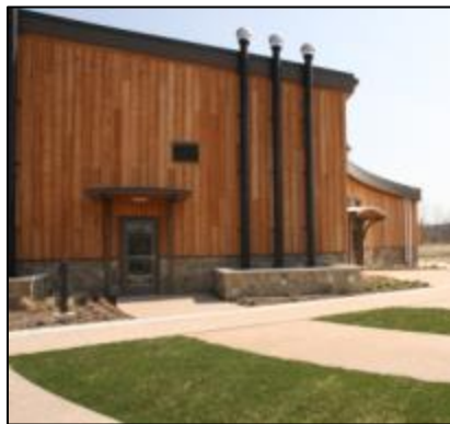
Ventilation System (stacks) for Waterless Sanitation System
