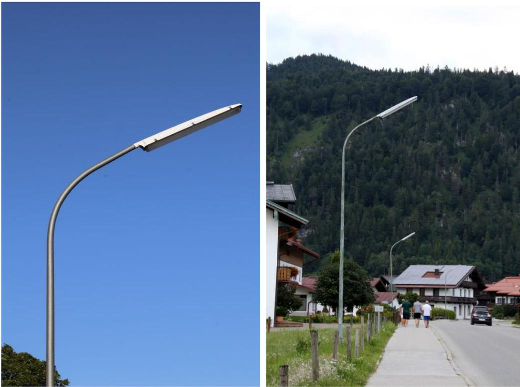
Fig. 17: The highly inclined luminaires (“Langfeldleuchte”) with fluorescent tubes. (photos: A. Hänel)
