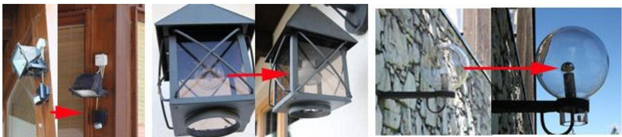
Fig. 14: Some examples of exchanges: changing inclination of floodlights, globe bulb to reflector bulb, globe bulb to top mirror bulb (photos *M. Philipp*)
