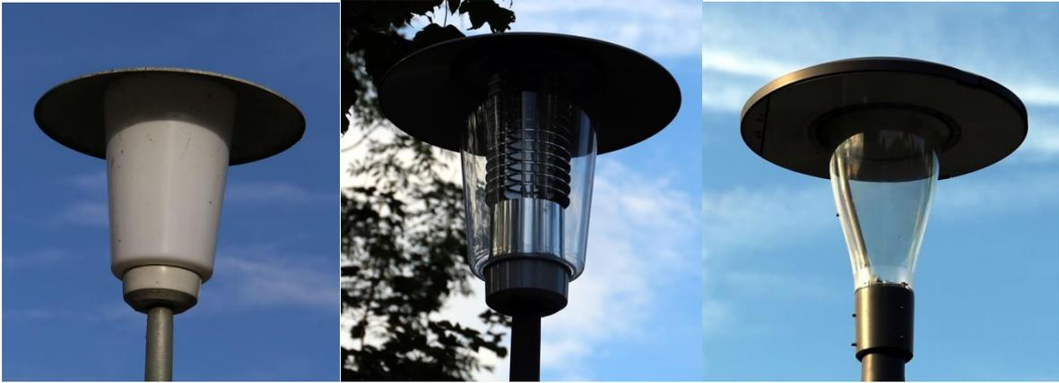
Fig. 19: Left: the traditional “mushroom” luminaires, middle: modern form with shadings and right: with LED. (photos: A. Hänel)
