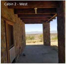
The position of the sockets under the porch covering makes it so they do not contribute to sky glow, however exposed bulbs create glare that is uncomfortable to the eye. Park management has committed to install shields for all exposed bulbs at each cabin within one year (May 2021).
